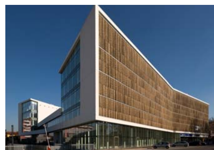
A sun protection system made of bamboo lamellae was applied mainly on the south facade.
